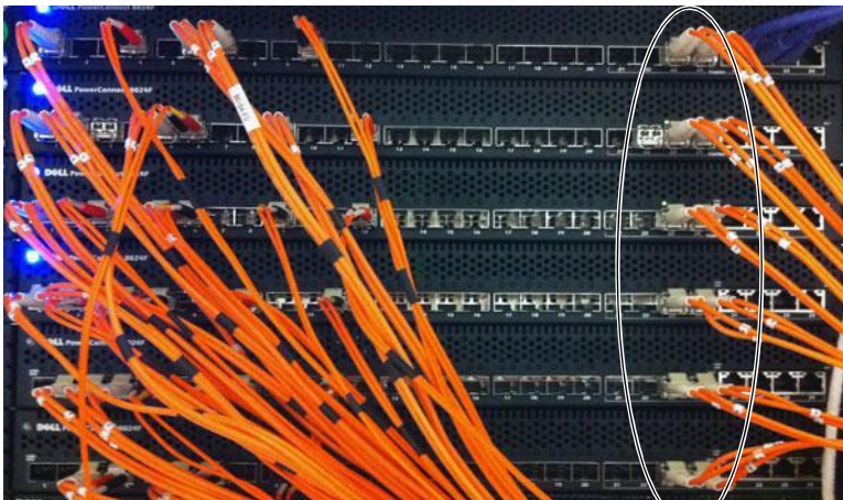
Figure 9-1. Connecting a Stack of PowerConnect 8024/8024F Switches
