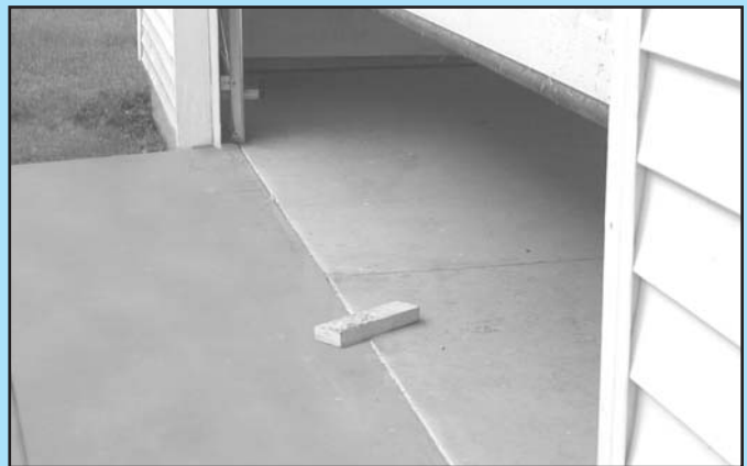
FIG. 6-5 2 x 4 under center of door opening.
